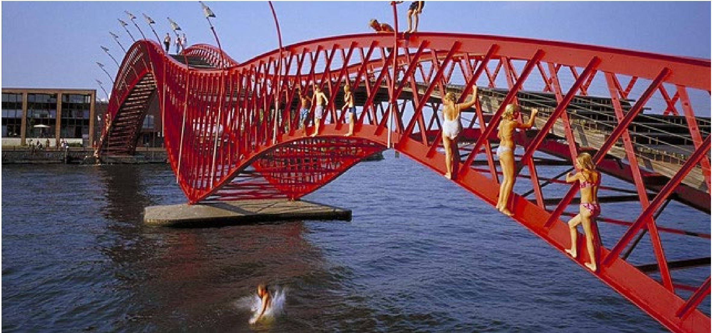
WEST 8 BRIDGES BORNEO-SPORENBURG 1998-2001, AMSTERDAM, THE NETHERLANDS
